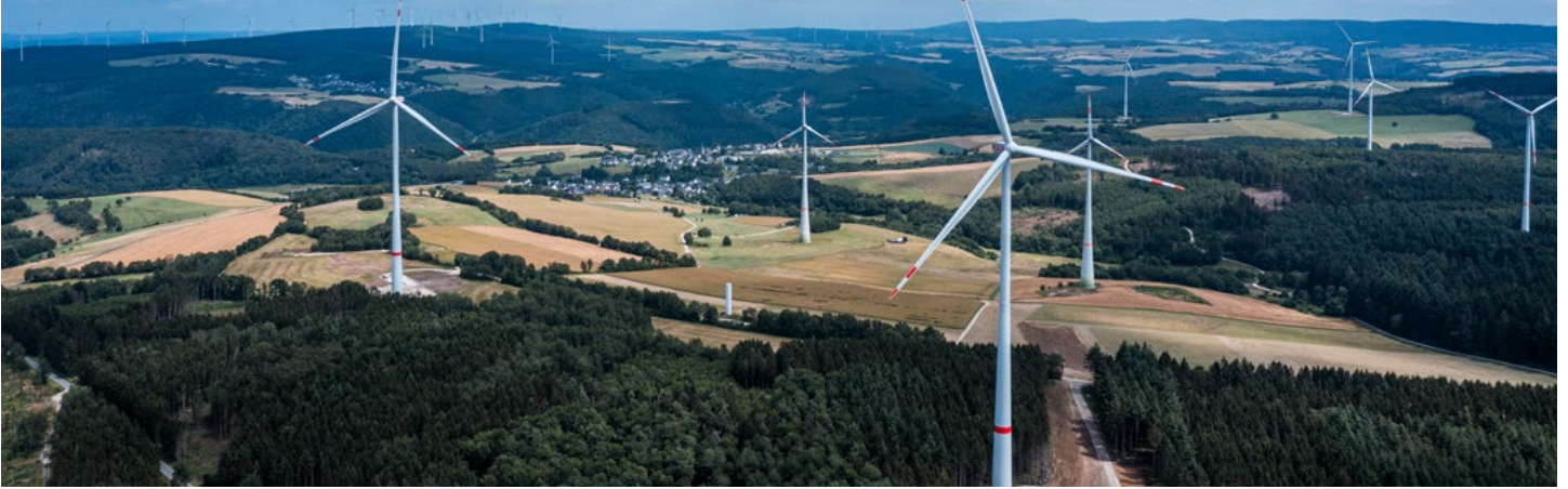
Tower segments from an old wind turbine are turned into a viewing tower that promotes tourism
