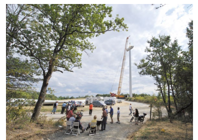
Construction of the Cuq wind farm in 2009
