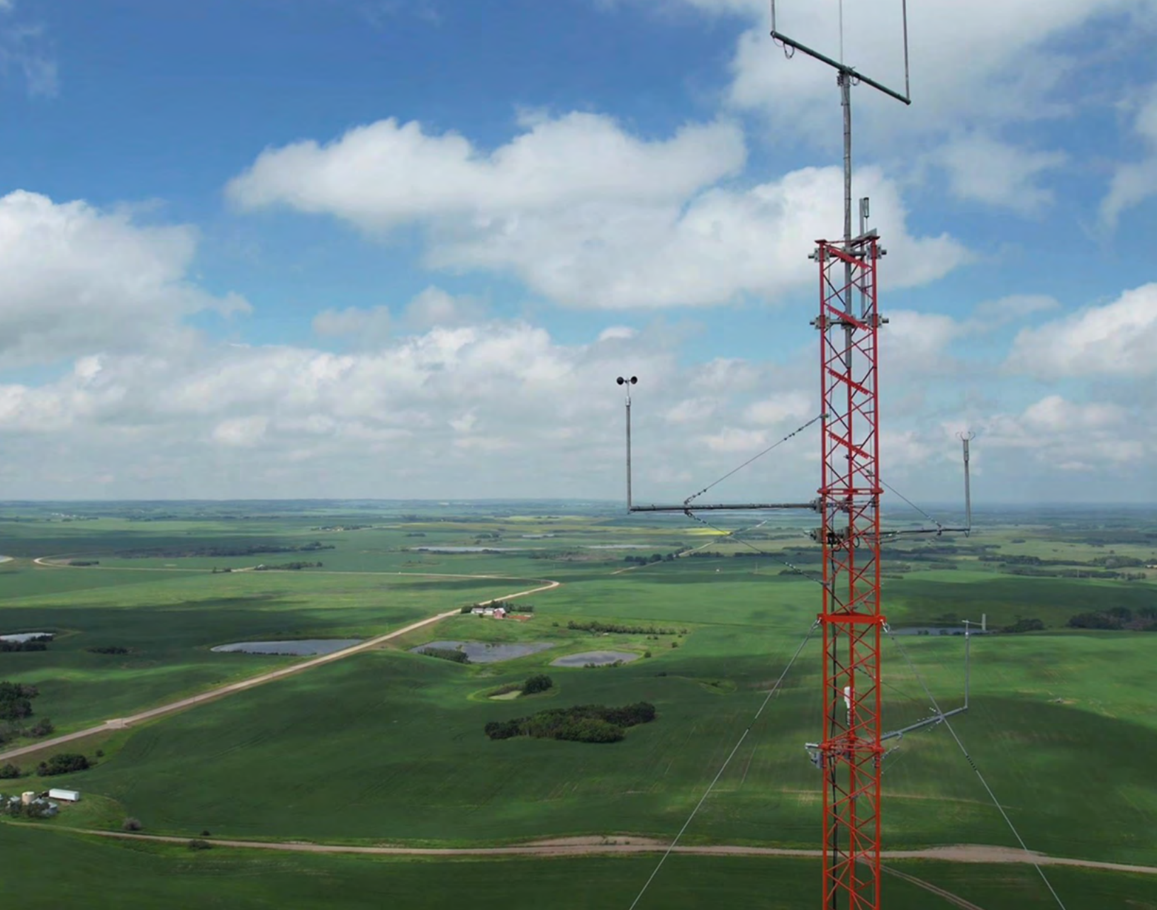
Project Meteorological Tower
