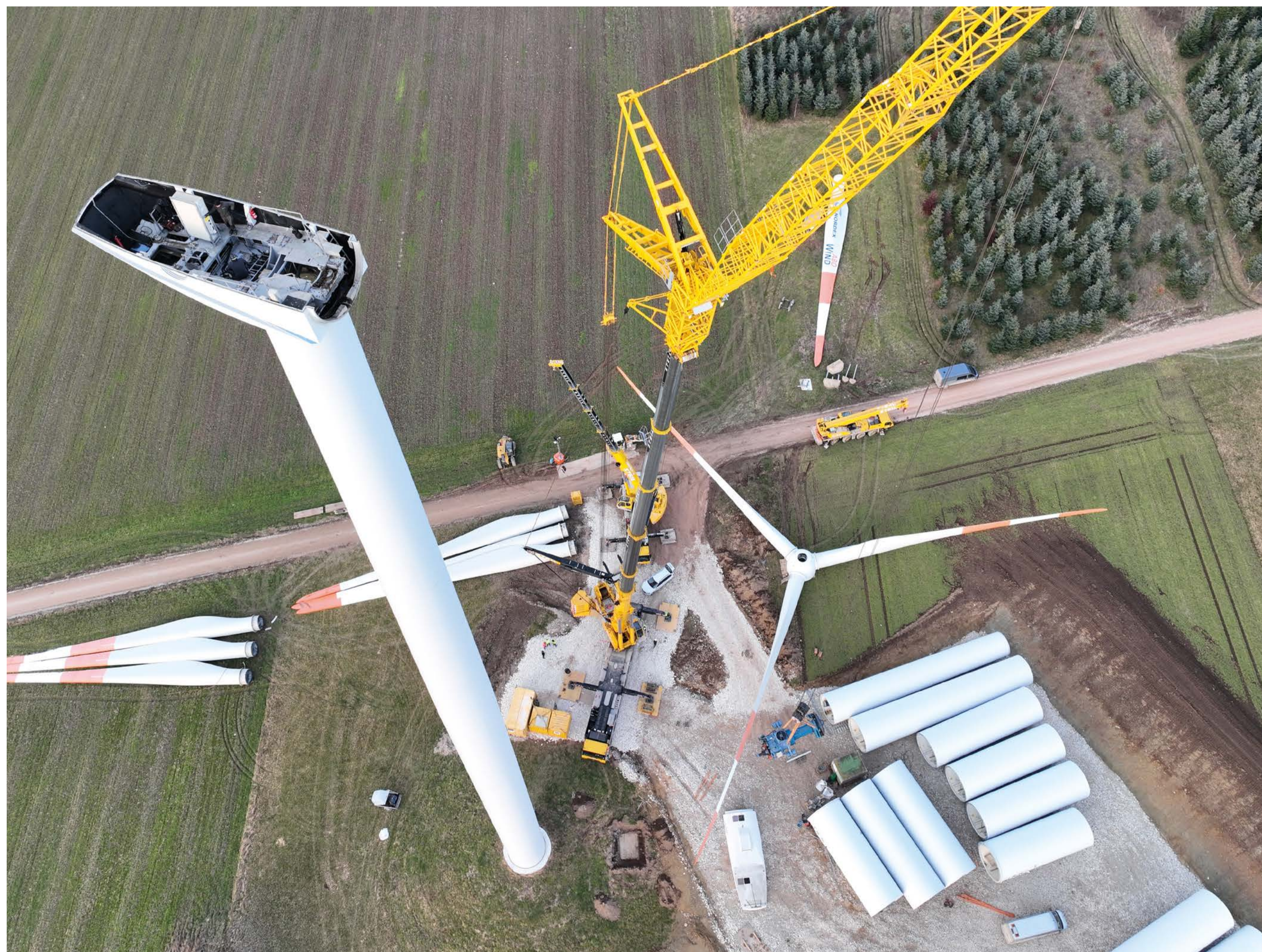
Dismantling wind farm
