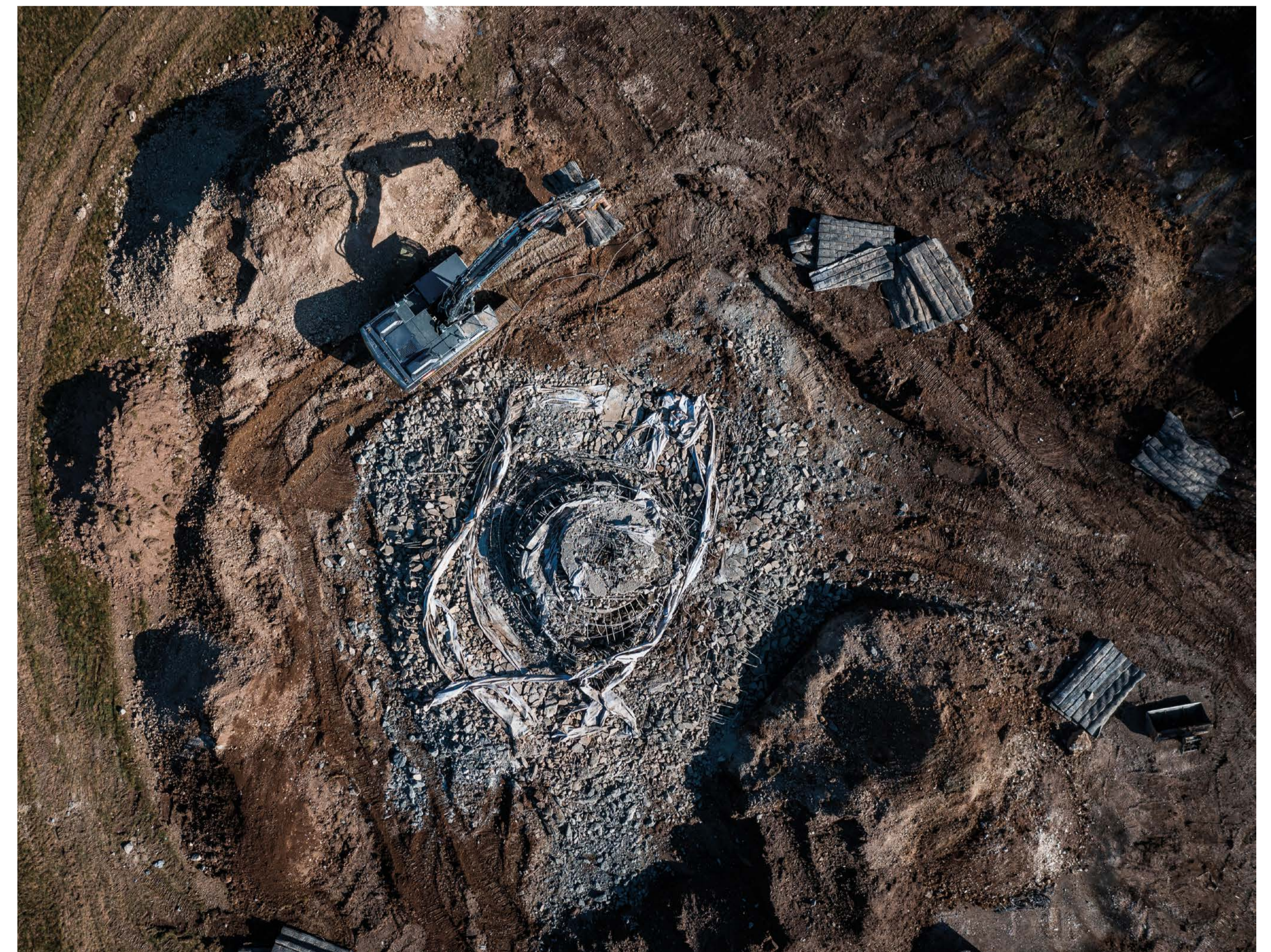
Deconstruction of foundation
