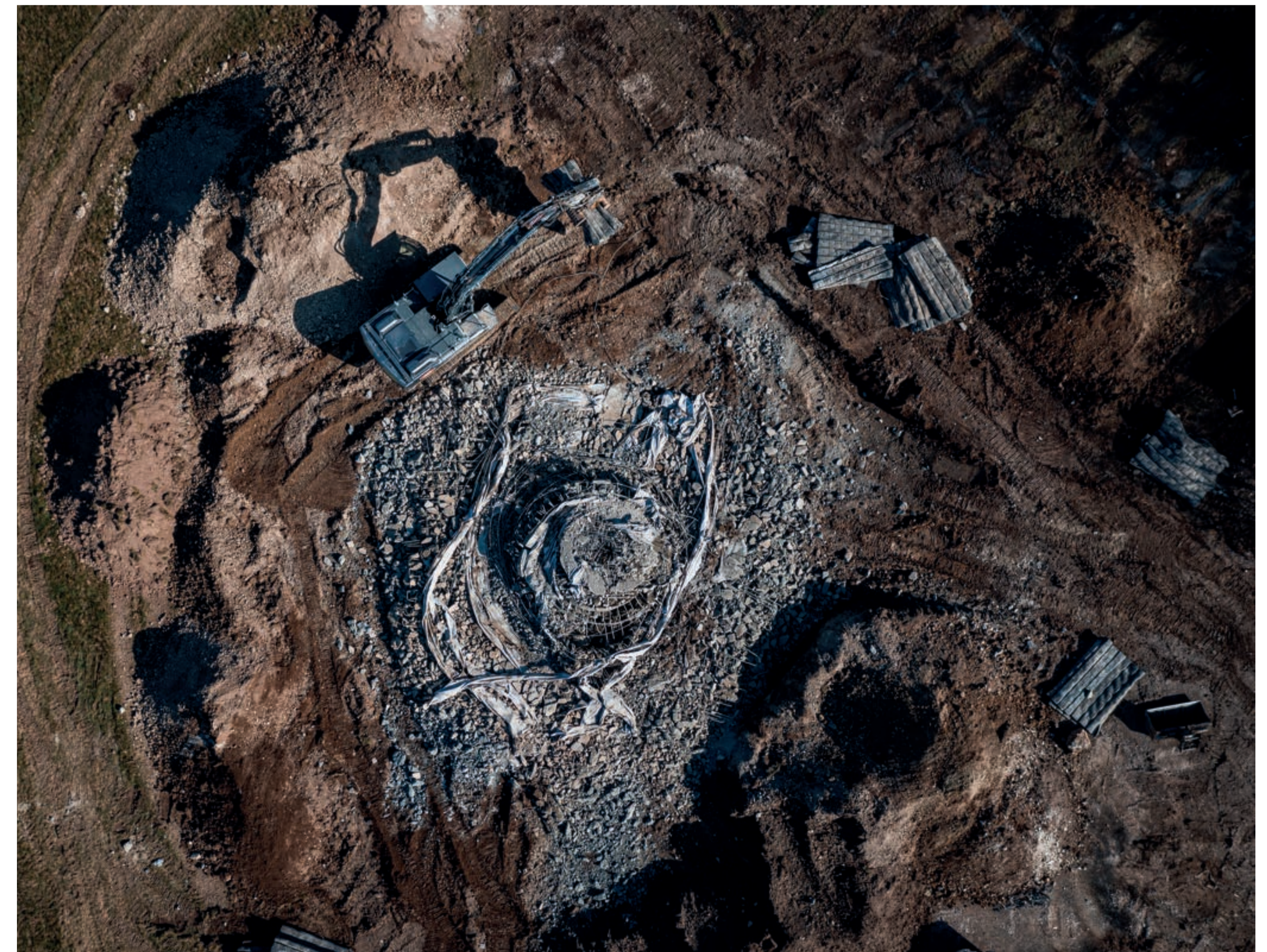
Deconstruction of foundation
