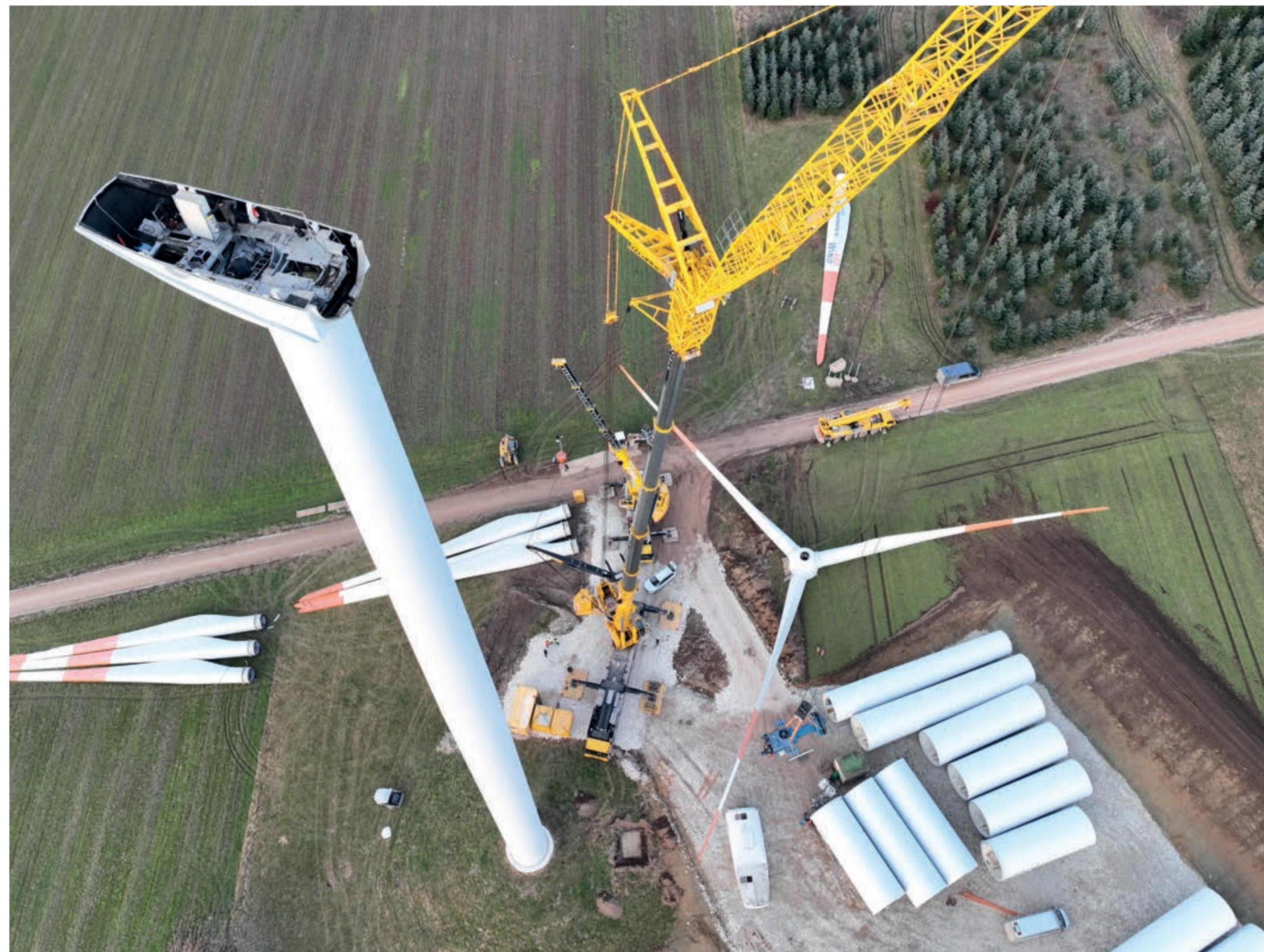
Dismantling wind farm
