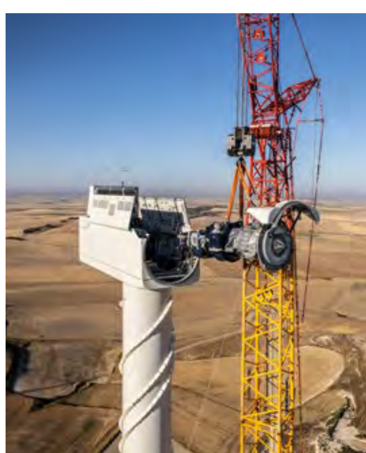
The drive rod is installed
