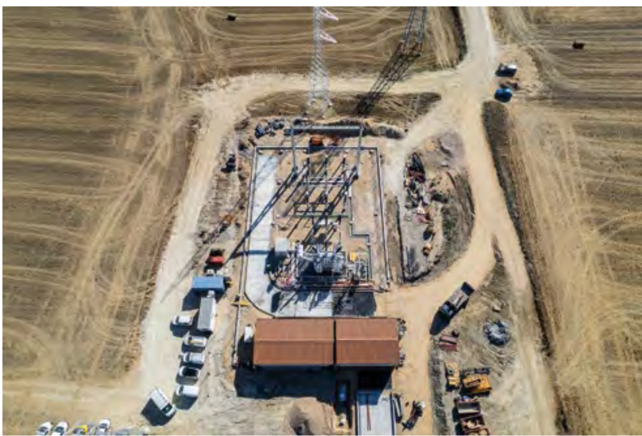
Construction of the transformer substation
