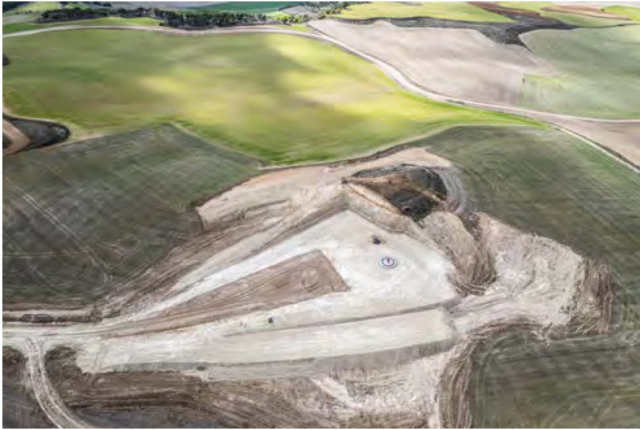
Ground movement on platforms
