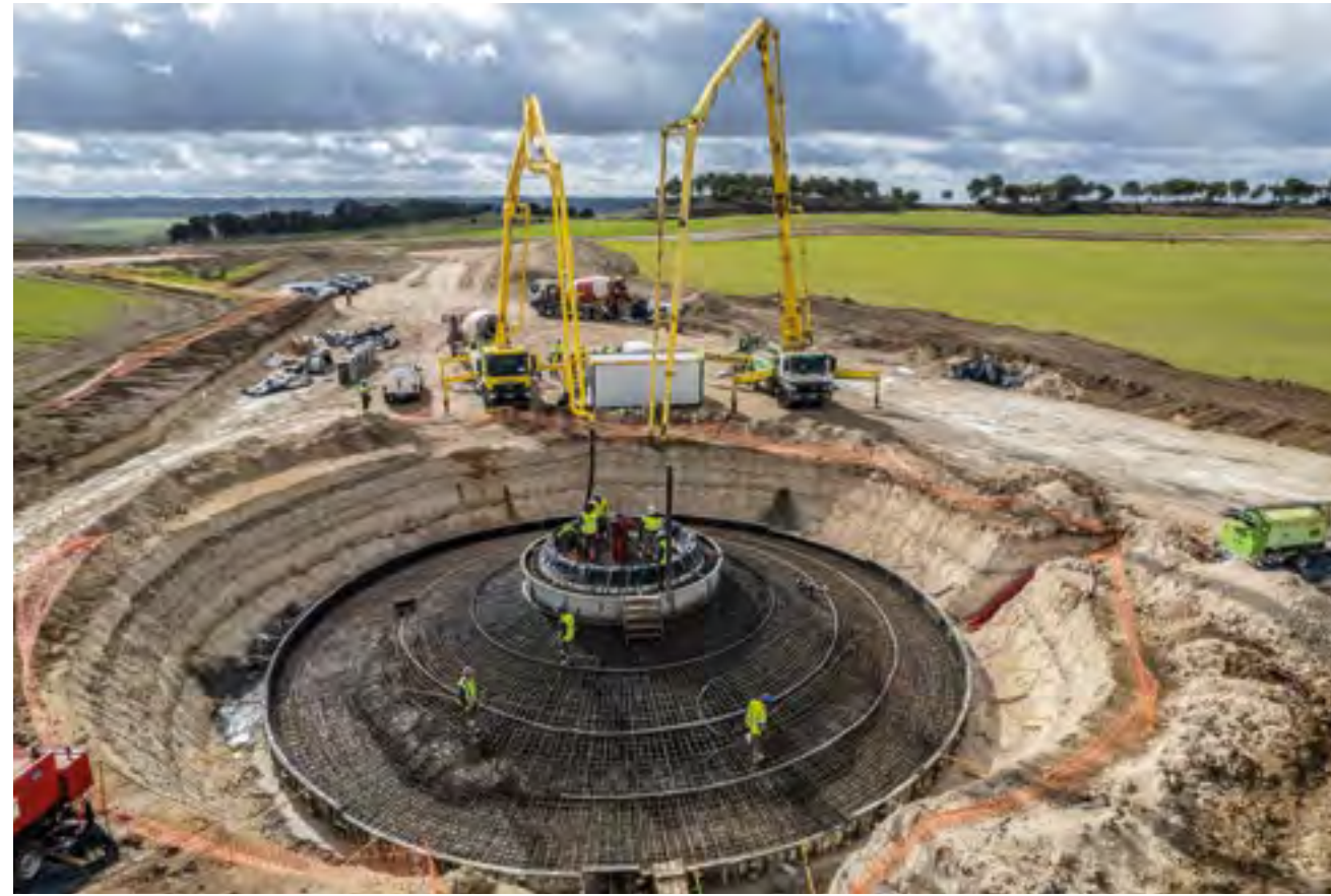
Construction of the foundation of a wind turbine base
