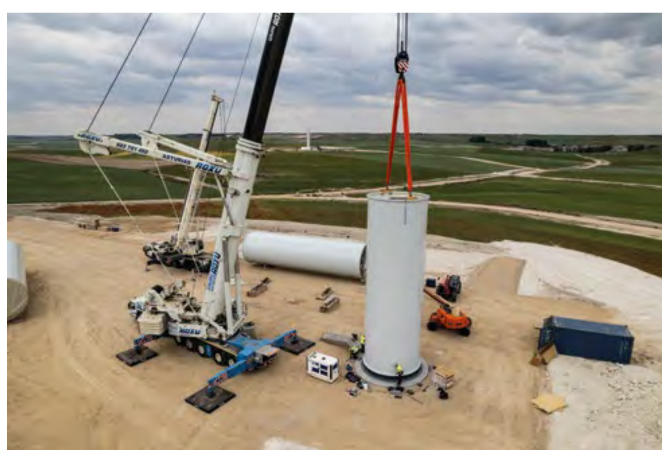
The first tower segment is bolted to the foundation
