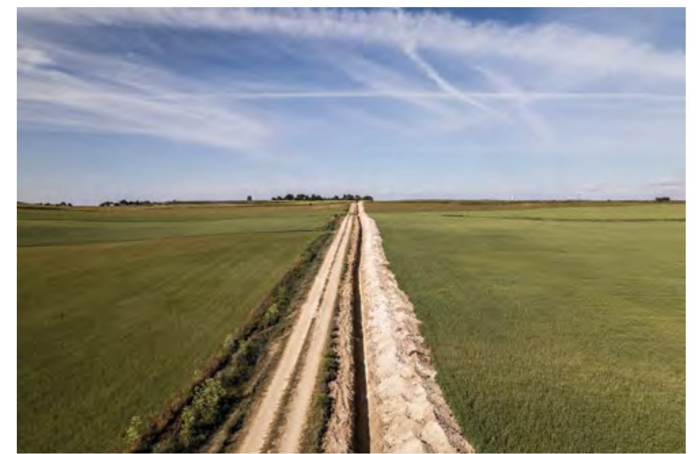
Trench for subway power line
