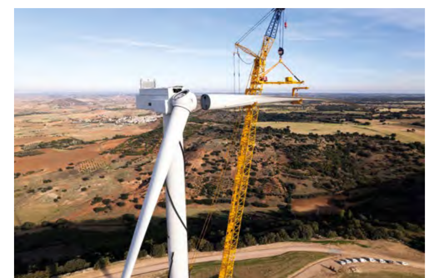
The three rotor blades are attached to the hub one after the other
