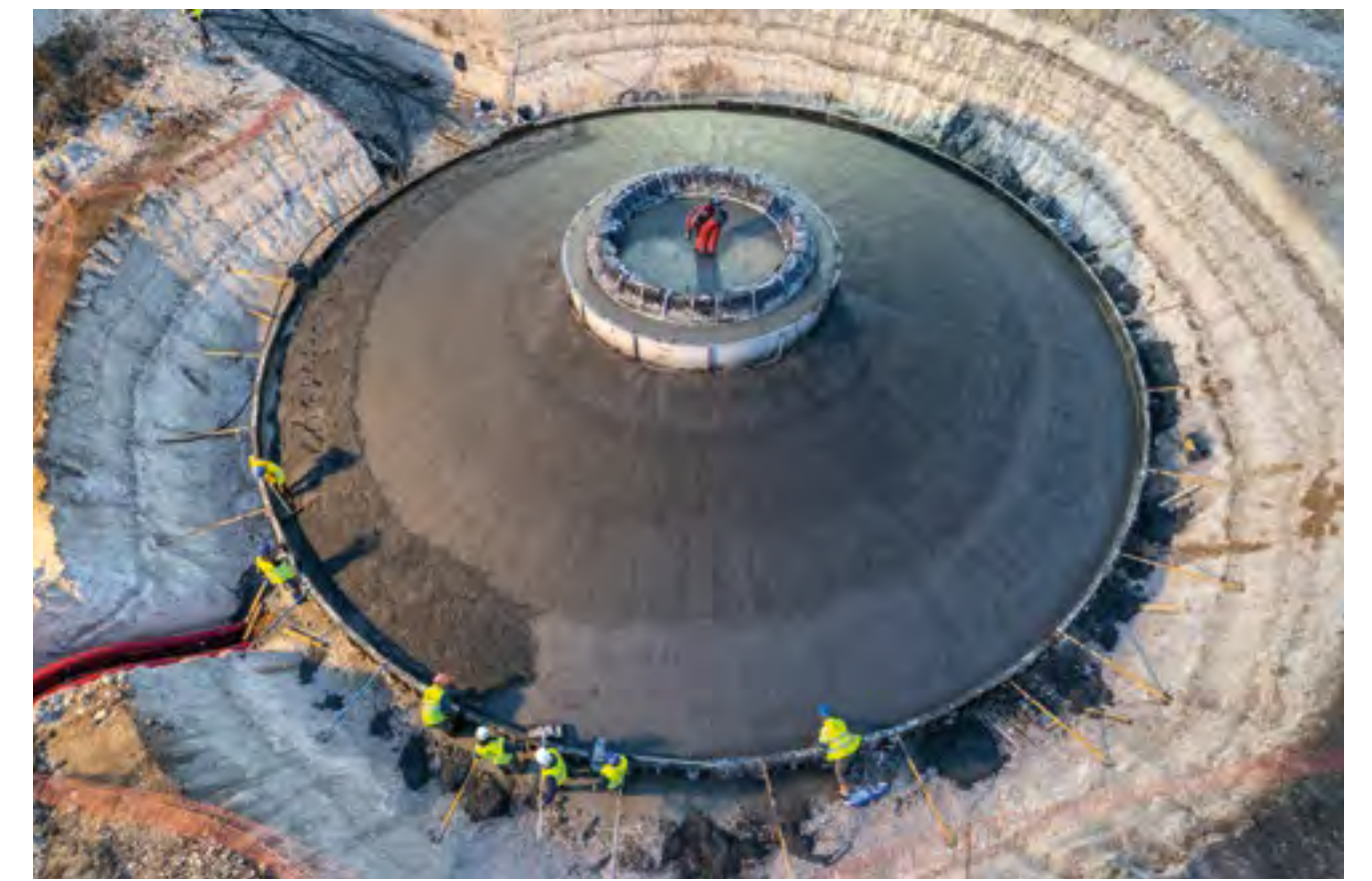
Concreting of foundations (500-600 m3 per wind turbine)
