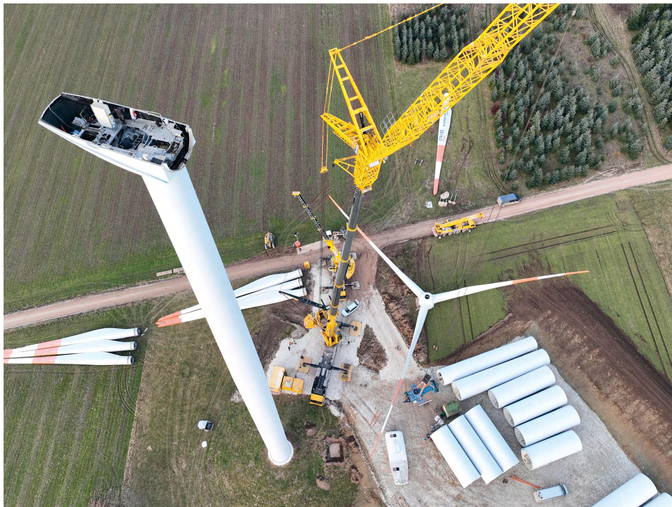
Dismantling wind farm
