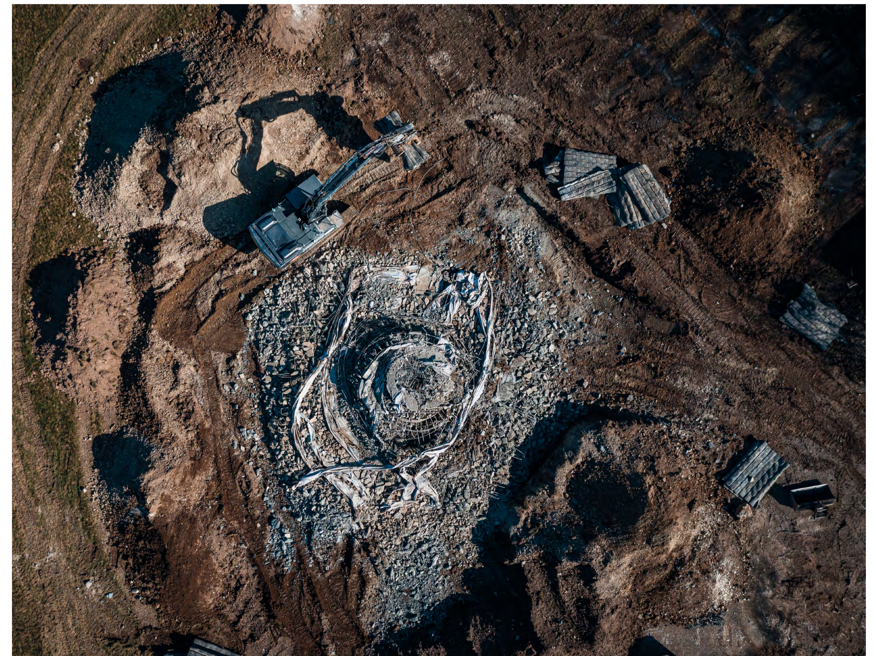
Deconstruction of foundation
