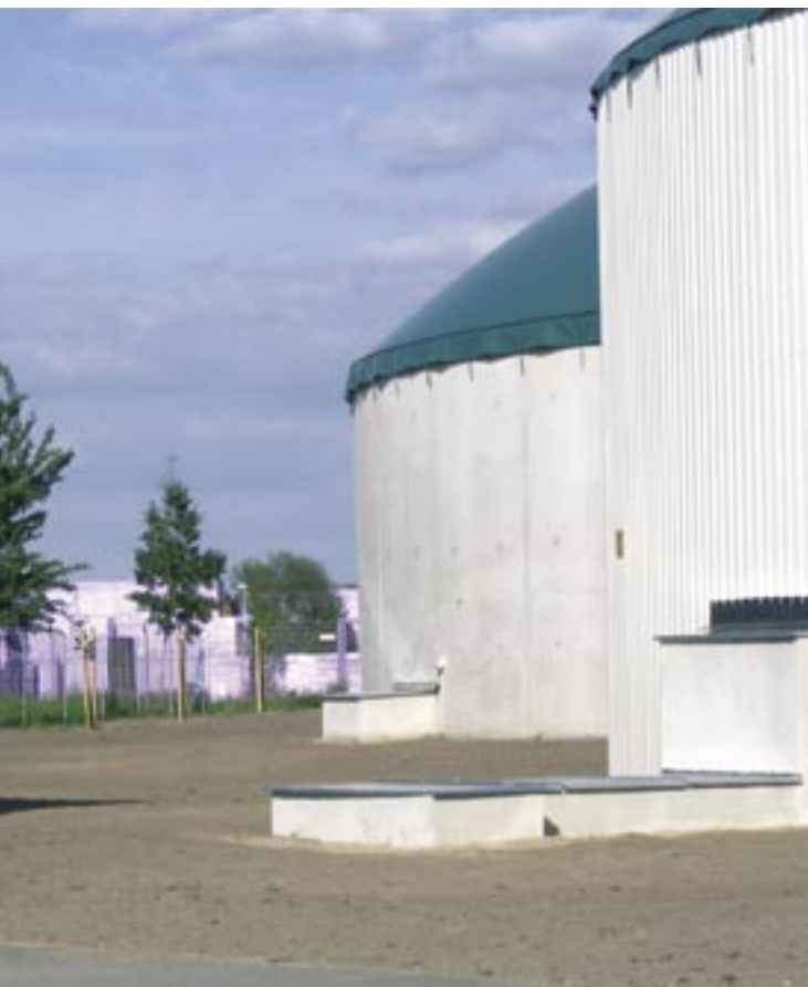
Biogasanlage Mechau / Mechau biogas plant
